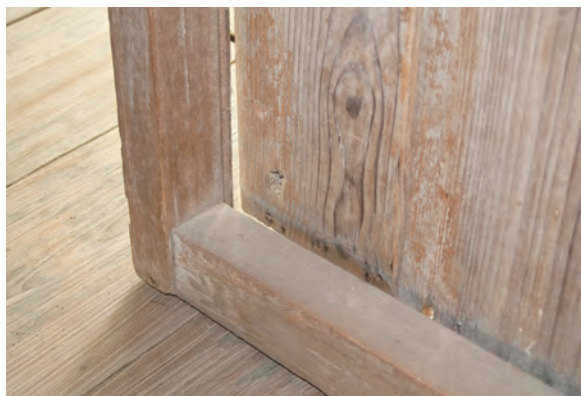
Figure 16. Current condition. Reverse side of painting of Shōki. The wooden planks of the door and the doorframe have become misaligned. Photograph collection of Chie Kyan. Permission of Ishigaki City Board of Education.
